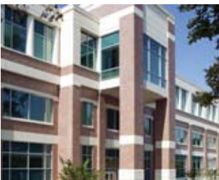
The precast insulated sandwich wall-panel system saved energy by increasing the R-value and eliminating thermal breaks.
