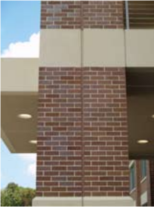
Exterior architectural finishes included thin brick and light-colored sand-blasted concrete.
