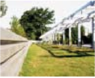
Georgia Institute of Technology is responsible for maintaining the landscaping on the Fifth Street Pedestrian Plaza Bridge in Atlanta, Ga. Courtesy of ARCADIS: John Bullock Photos.
